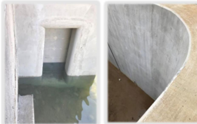
Photo 1.d. Fishway entry flush with floor with rounded edges and 6" radius. Fishway walls were rounded for lamprey movement and to reduce turbulence
