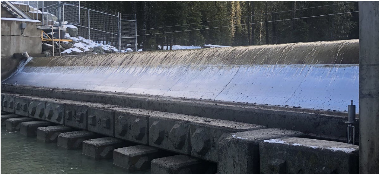
Figure A-6. Example of a Coanda screen (photo from Elgin Separation Solutions; https://elginseparationsolutions.com/coanda-screens/ )
