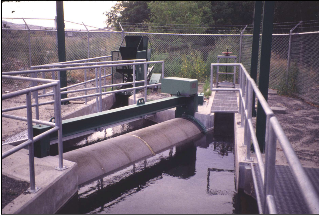
Figure A-1. Example of a drum screen facility.
