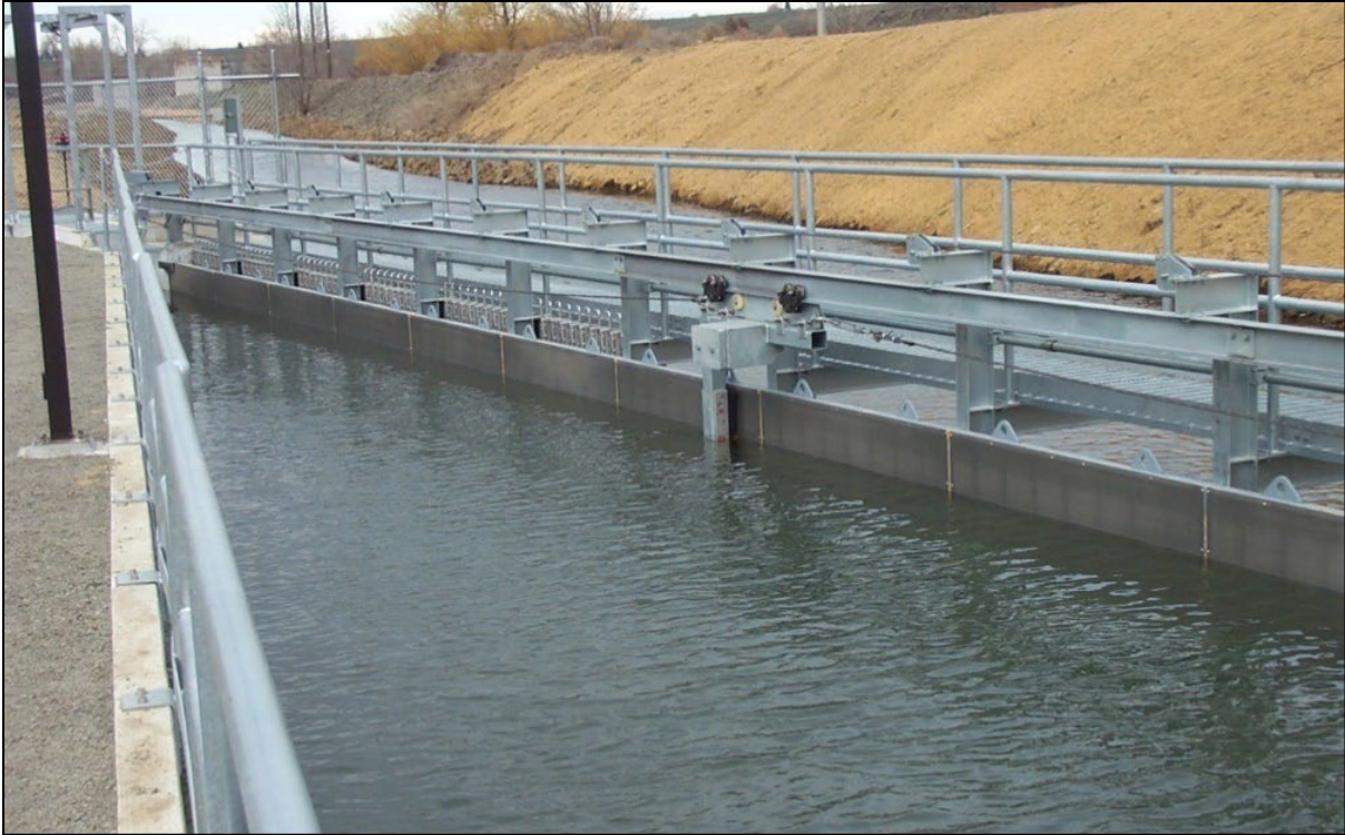
Figure A-3. Example of a vertical flat plate fish screen facility with a gang brush cleaning system.
