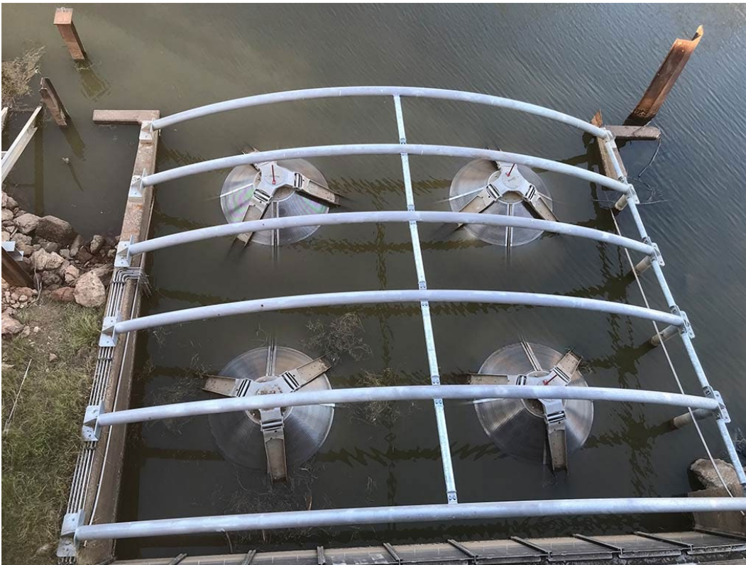
Figure A-2. Example of a cone screen facility (photo from awma Water Control Solutions; awmawatercontrol.com.au ).
