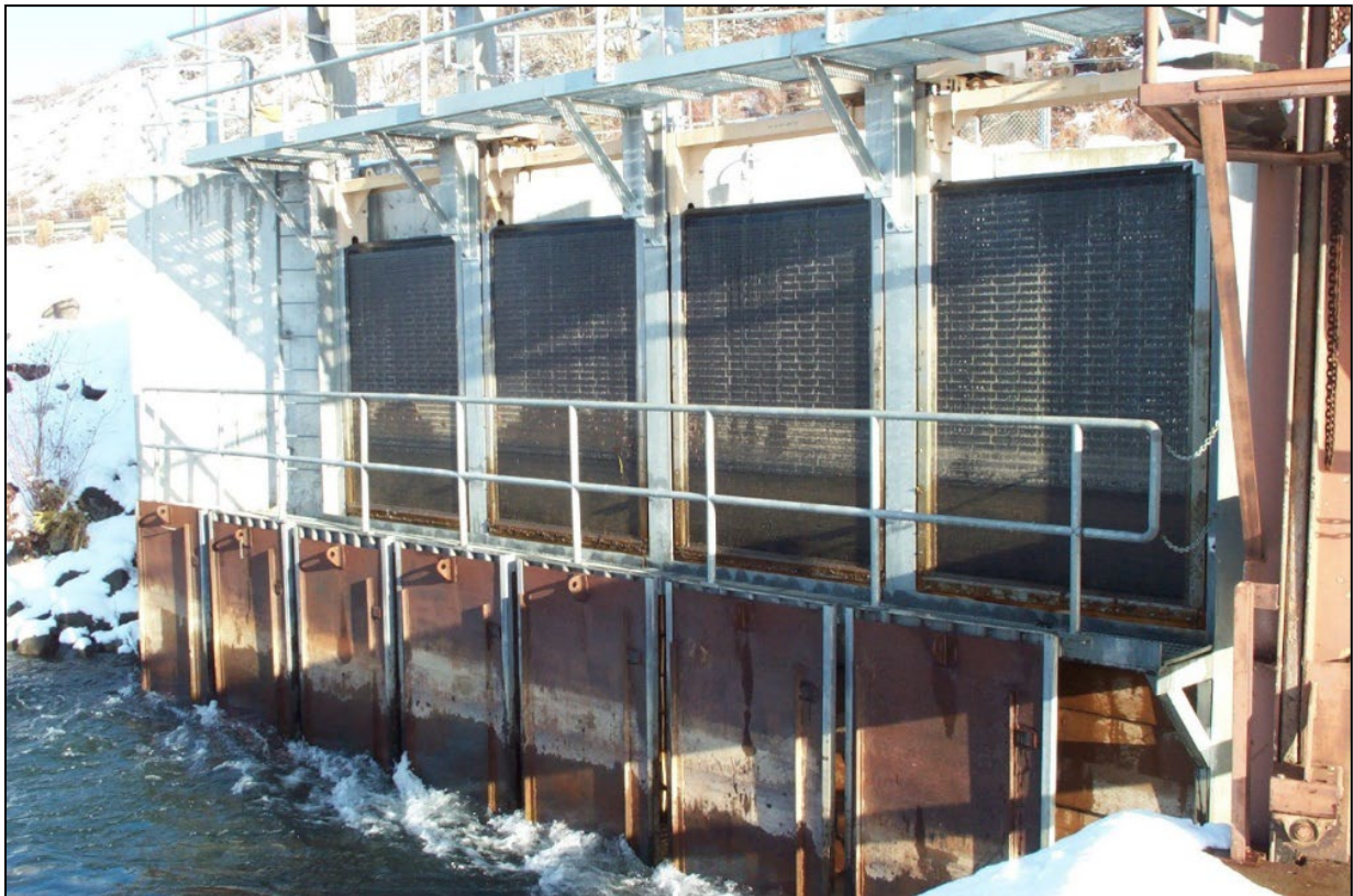
Figure A-4. Example of a belt screen facility.
