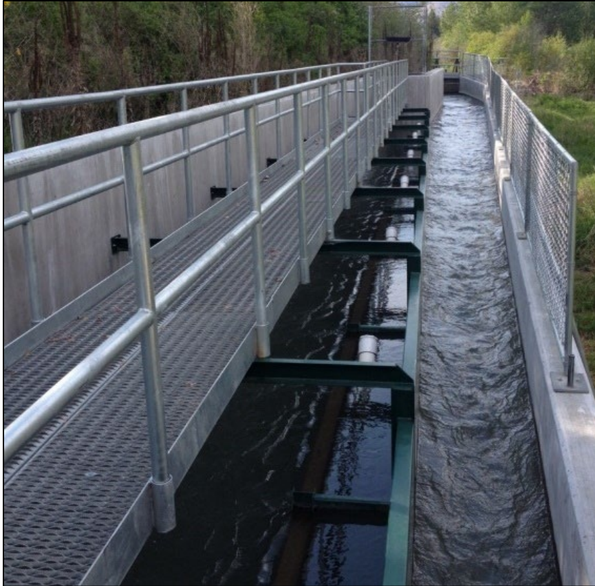
Figure A-5. Example of a horizontal fish screen
