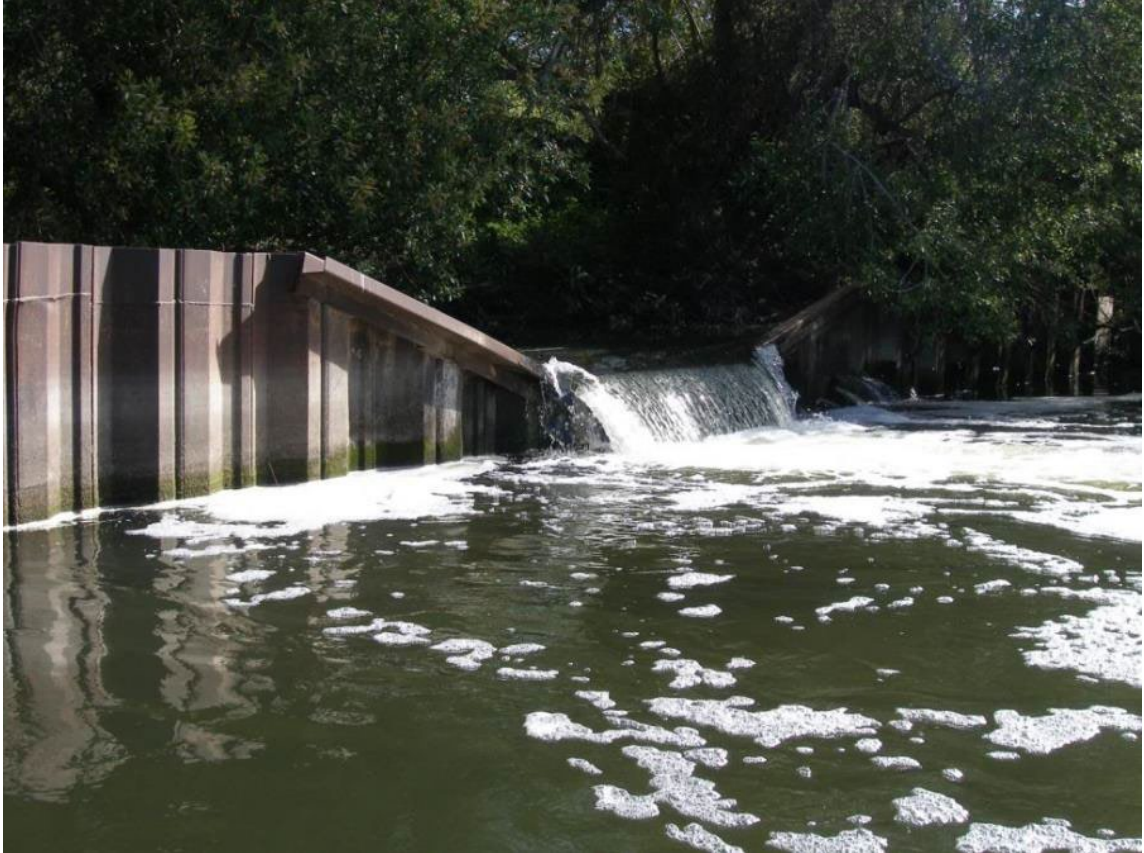
Figure 11. The Marre Tidal Weir at the San Luis Obispo Creek estuary. The weir was modified in 2006 to provide improved passage for coastal Rainbow Trout. Unfortunately, the design likely excluded Pacific Lamprey and may have extirpated the population. However, a new lamprey passage structure was installed in 2013 and lampreys recolonized the drainage by 2017 (Reid and Goodman 2020). Photo taken in March 2012.
