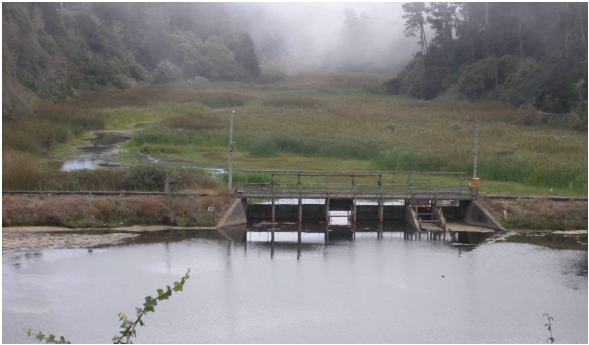
Figure 4. Dam and fish ladder in the estuary of Pudding Creek. This location was used to provide water to a neighboring lumber mill that is no longer in operation. It now serves as a fish population monitoring facility. No records of Pacific Lamprey exist for Pudding Creek and they do not currently occupy the drainage. Improving passage at the fish ladder may improve the potential for future colonization.
