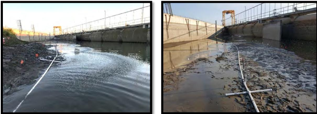
**Figure 5.7.** Overview of the sprinkler water system operation upstream of the fish screens at Wapato Diversion immediately after dewatering of key larval lamprey habitat occurred (left photo). In the right photo, the sprinkler water system is laid down on the flat surface where many larvae remain after dewatering.
