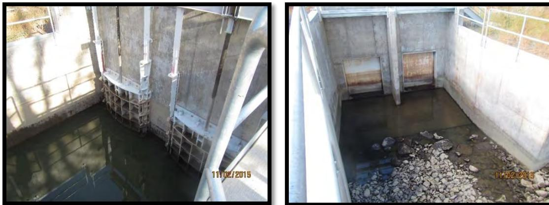
**Figure 6.30.** The regulating gates after dewatering looking downstream (left photo). The regulating gates after dewatering looking upstream (right photo). In 2018, the gates were fully shut after the reopening of the headgates for the winter months. Water level is generally low after irrigation shutdown, limiting potential damages caused by freezing water coming into contact with the gates.
