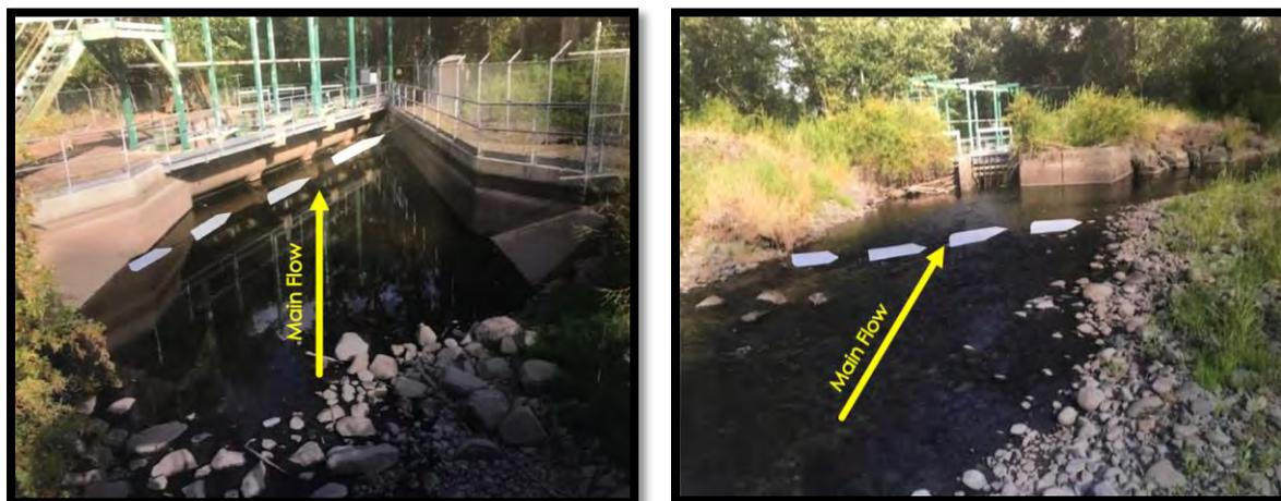
**Figure 6.36.** Overview of the planned placement locations for the FVES units at Bachelor-Hatton Diversion. The left photo shows the thalweg flow (yellow arrow) immediately upstream of the fish screens, and planned directed flow by the FVES unit at this location. The right photo shows the thalweg flow (yellow arrow) immediately upstream of the headgate, and the planned flow direction by the FVES unit at this location.
