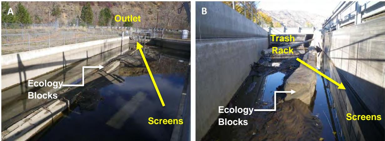
**Figure 7.7.** (A) Ecology blocks laced downstream of the drum screens at Town Diversion, effectively capturing fine sediment that would have otherwise traveled down the canal. (B) Ecology blocks placed upstream of the vertical screens at Naches-Selah Diversion, preventing fine sediment to collect in front of the fish screens. Yellow arrow shows the direction of water flow.
