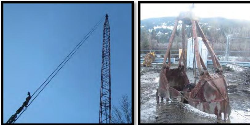
**Figure 4.11.** The 150-ft tall crane (top photo) and the dredge grabber (bottom photo) used for the dredging operation at Dryden Diversion forebay.
