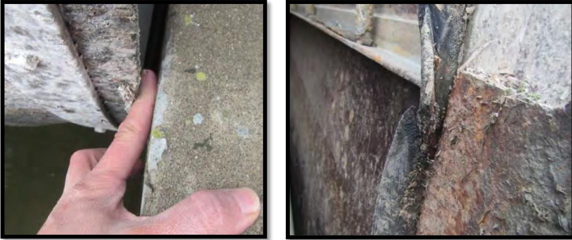
**Figure 6.11.** Examples of gaps/tears observed at Sunnyside Diversion during winter of 2013. The size of gaps ranged from 5-14 mm. The left photo shows a gap with a 14-mm opening. The right photo displays a damaged rubber seal, resulting in a larger opening.
