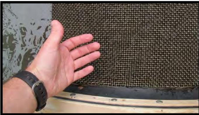
**Figure 3.23.** Woven wire mesh with a 3/32" (2.84 mm) opening at Congdon Diversion.
