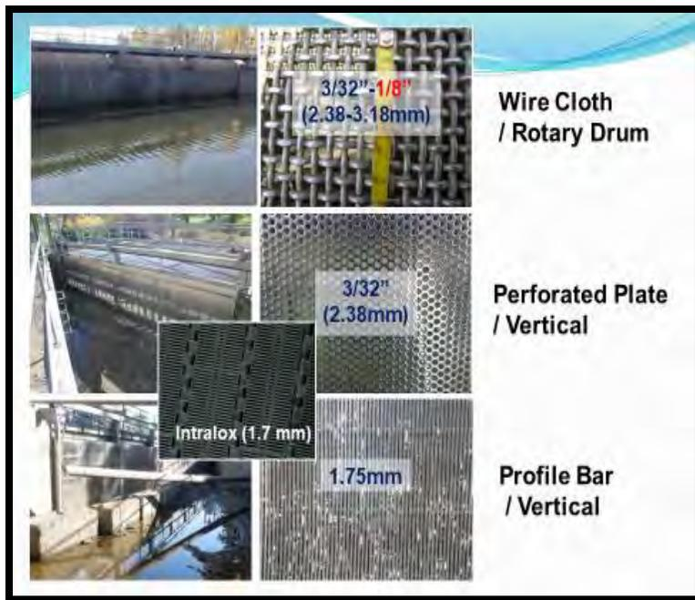
**Figure 6.3.** Photos displaying the four main types of screens and examples of facilities that use these screens. The NOAA Fisheries salmonid criteria for the mesh opening size are also displayed for each screen type.
