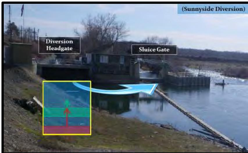
**Figure 7.6.** Diversion headgates that open from mid-water column (green area) rather than the bottom (red area) will likely help reduce entrainment for lampreys that congregate in the forebay upstream of the headgate, such as at Sunnyside Diversion shown here. Opening sluice gates prior to the start of the irrigation season during high flow events should also help move the larvae congregating in the forebay and minimize their entrainment into diversions.
