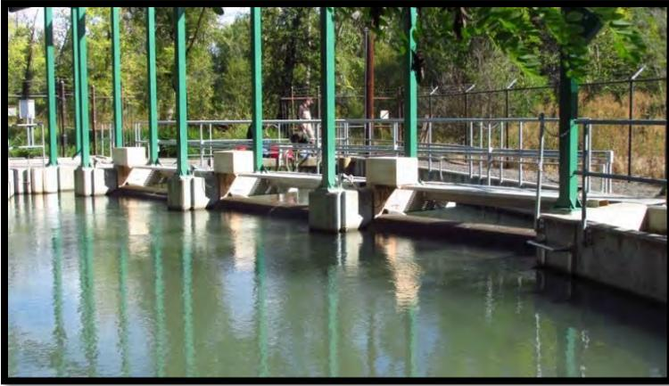
**Figure 3.22.** Looking upstream towards the three rotary drum fish screens at Condon Diversion.
