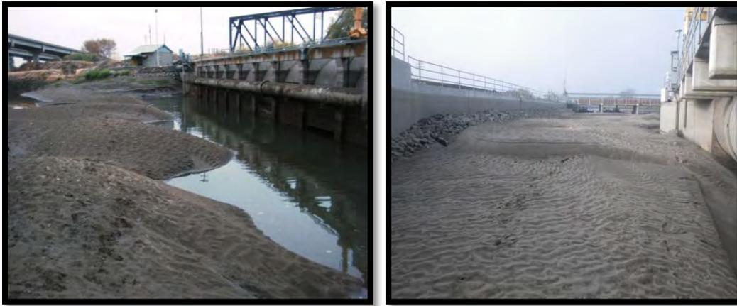
**Figure 6.22.** Examples of diversions with a high accumulation of fine sediment accumulation. Left photo shows the sediment accumulation at Sunnyside Diversion (Yakima River, Union Gap, WA) downstream of the fish screens after dewatering. The right photo shows the built-up of sediment at Chandler Diversion (Lower Yakima River, Prosser, WA) immediately upstream of the fish screens after dewatering.
