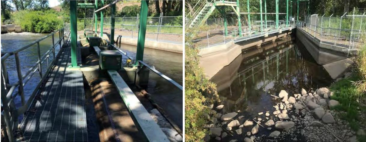
**Figure 6.34.** Overview of Bachelor-Hatton Diversion on Ahtanum Creek. The left photo shows the diversion with water flowing during the irrigation season (flow from left to right). The right photo shows the area upstream of the fish screens after dewatering in July, 2018 (photo taken from the headgate facing downstream).
