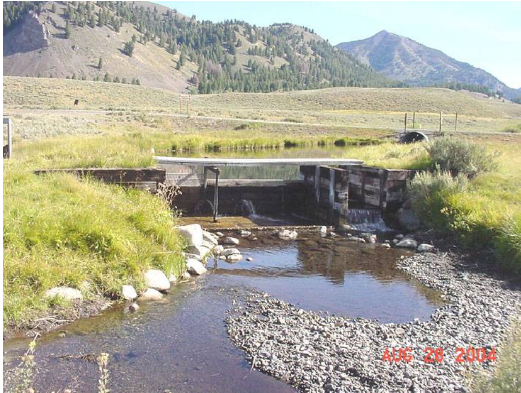
Figure 9. Irrigation diversion that blocks upstream movement, entrains lamprey and other fish into the ditch, and dewateres downstream reaches.
