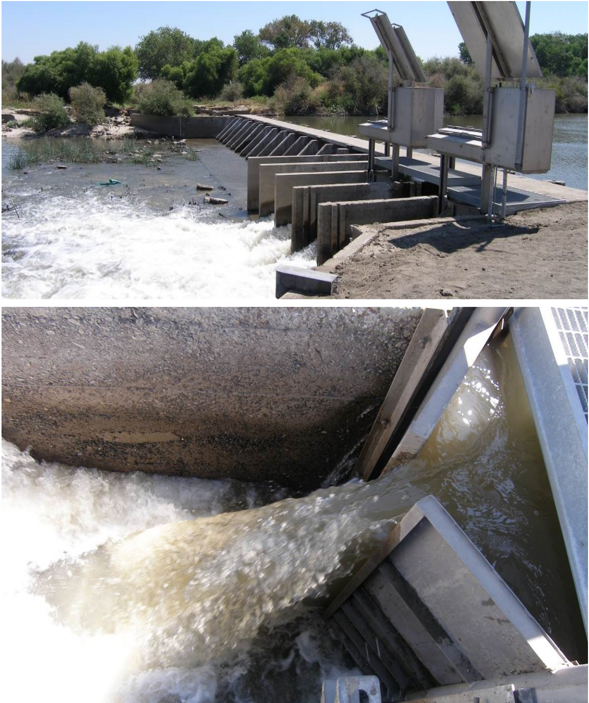
Figure 7. Sack Dam on the San Joaquin River near Los Banos (top) and hydraulic conditions within one gate (bottom). This site is currently an obstacle to upstream migration of adult lampreys. The dam provides water through an unscreened diversion to the Arroyo Canal which may entrain downstream migrant lamprey. Constructing a fishway over Sack Dam and screening the Arroyo Canal diversion are actions that will be accomplished by the San Joaquin River Restoration Program.
