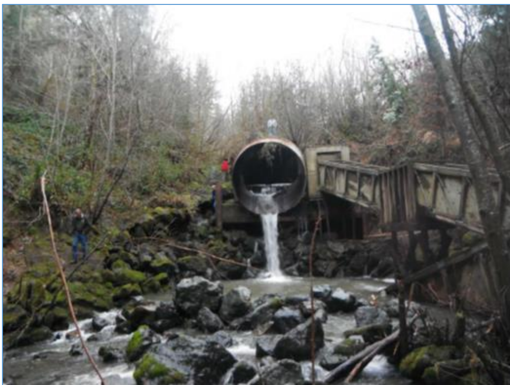
Photo 1 – Baker Creek culvert during winter low flow.
