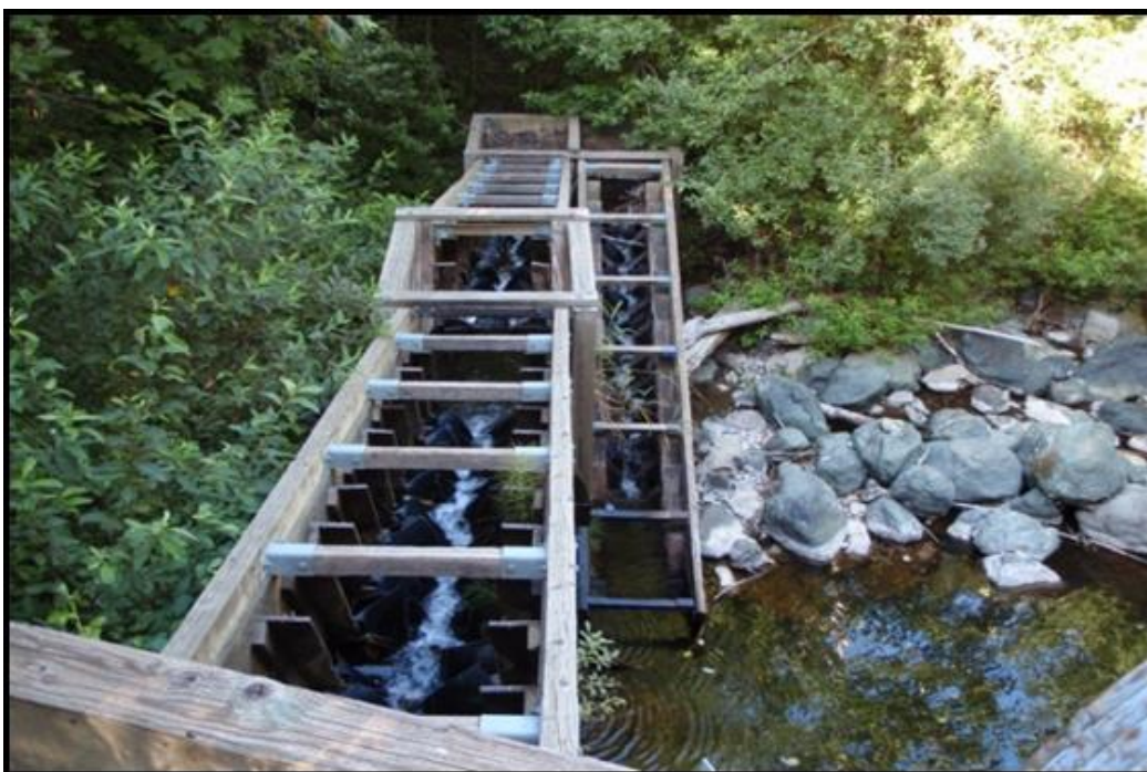
Photo 2 – Denil fishway during summer low flow.
