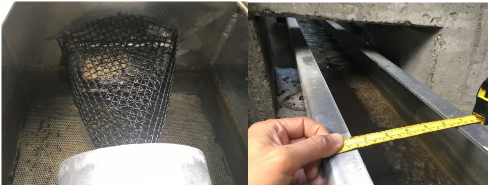
Figure 2. The resting box (left photo) for the Lamprey Passage Structure at Lyle Falls Dam. With some modification, adult lamprey could potentially be trapped here daily and PIT tagged to evaluate passage at Lyle Falls and within the fish ladder (to determine the best way to increase passage here).
