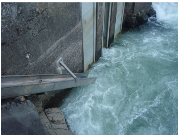
Figure 3. The Lyle Falls LPS is perched during low flow season, often preventing adult lamprey from using it during the key migration period in the summer (July-September)
