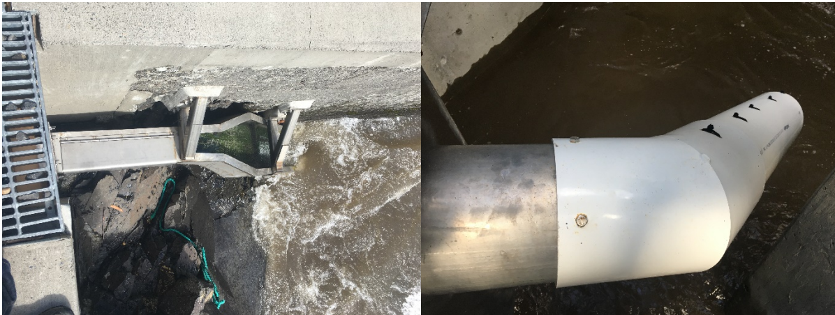
Figure 1. Lamprey Passage Structure at Lyle Falls Fish Ladder. The entrance of the LPS is in a great location, but the volitional release point is currently at the bottom of the fish ladder (inhibiting passage of adult lamprey if they struggle within the fish ladder).
