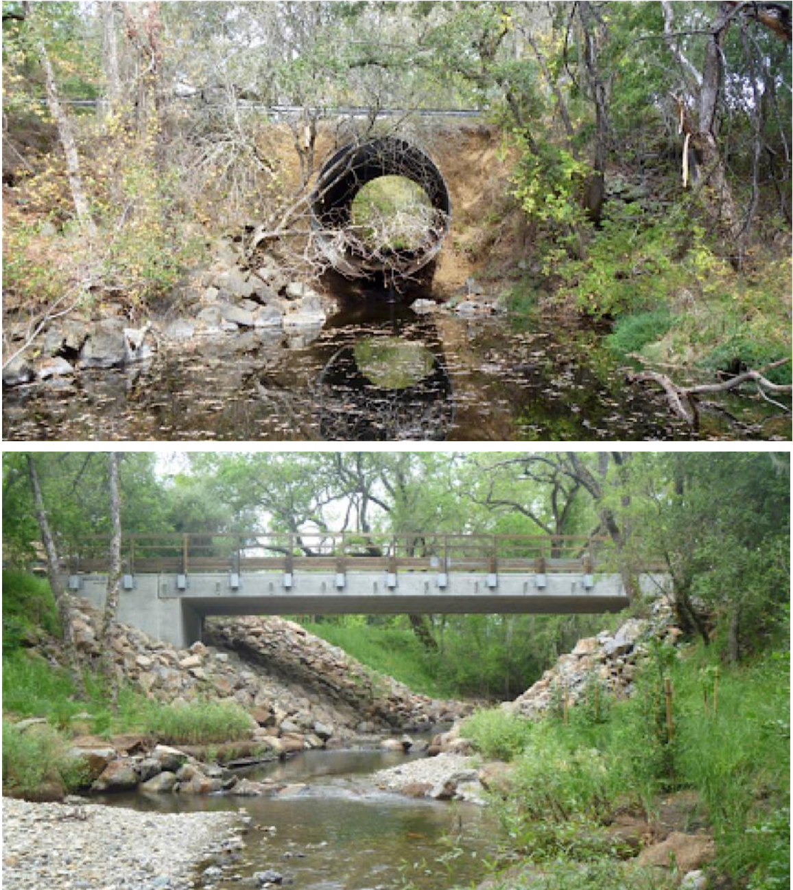
Figure 5. The Greenwood Road culvert was initially identified as a total barrier to Pacific Lamprey on mainstem Napa River, although resident brook lamprey occur upstream, indicating habitat suitability. The culvert was removed in 2015 by NRRCD and replaced by a bridge, opening access to 2.75 mi of habitat below Kimball Canyon Dam.
