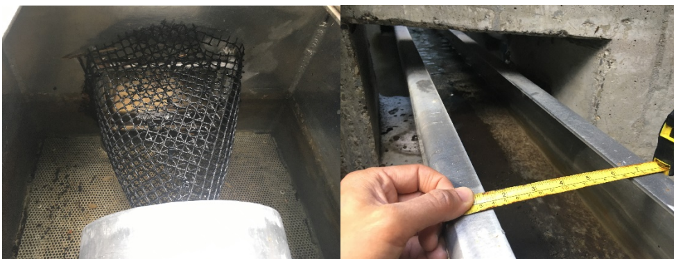
Figure 3. The resting box (left photo) for the Lamprey Passage Structure at Lyle Falls Dam. With some modification, adult lamprey could potentially be trapped here daily and PIT tagged to evaluate passage at Lyle Falls and within the fish ladder (to determine the best way to increase passage here).
