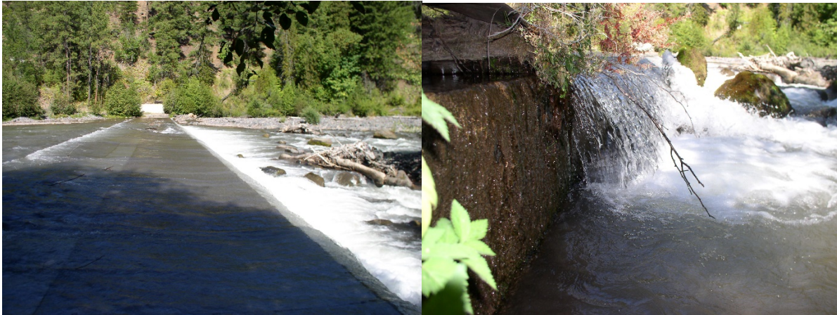
Figure 1. Klickitat Hatchery weir during low flow period. The channel spanning edge/lip is 90 degree angle making it difficult for Pacific Lamprey to climb.
