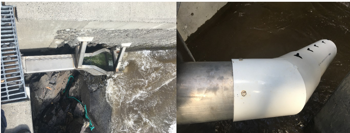
Figure 2. Lamprey Passage Structure at Lyle Falls Fish Ladder. The entrance of the LPS is in a great location, but the volitional release point is currently at the bottom of the fish ladder (inhibiting passage of adult lamprey if they struggle within the fish ladder).
